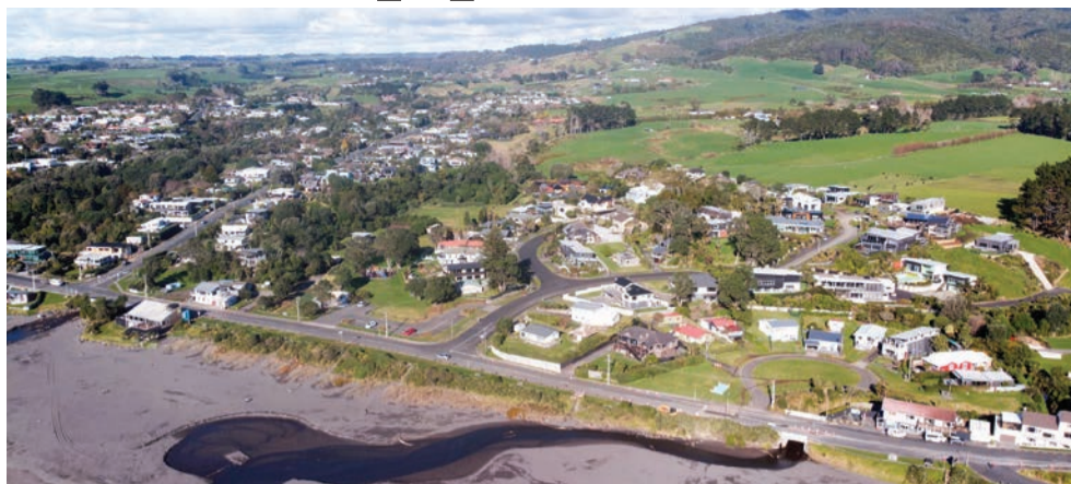
Water projects in Oākura include a new bore and upgrades to the Oākura Water Treatment Plant.
